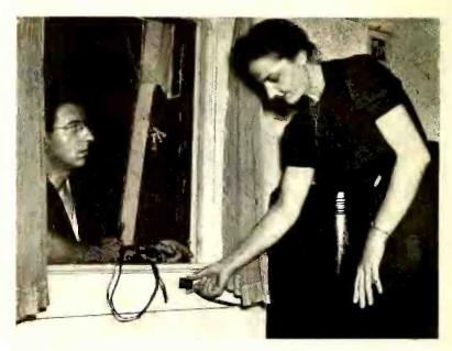
Handy wall outlet installed at the window eliminates messy and trouble-some antenna and ground lead-in wires. This unit offered by Cornish some antenna and ground lead-in wires. This unit offer Wire is easily installed by the serviceman.
